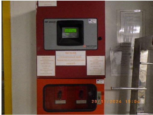
Fire Alarm Control Panel
